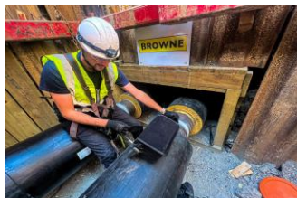
Figure 1 Installation of twin 450mm DH pipes
