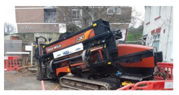
Disruption to local residents and the general public who use the footpath was kept to a minimum with this section of work being completed over a 10 day period. The no-dig solution ensured that only the entry and exit points for the drilling required re-instatement at street level. The actual footpath and grassed verge were untouched during the works, ensuring the aesthetics of the area remained unchanged.
