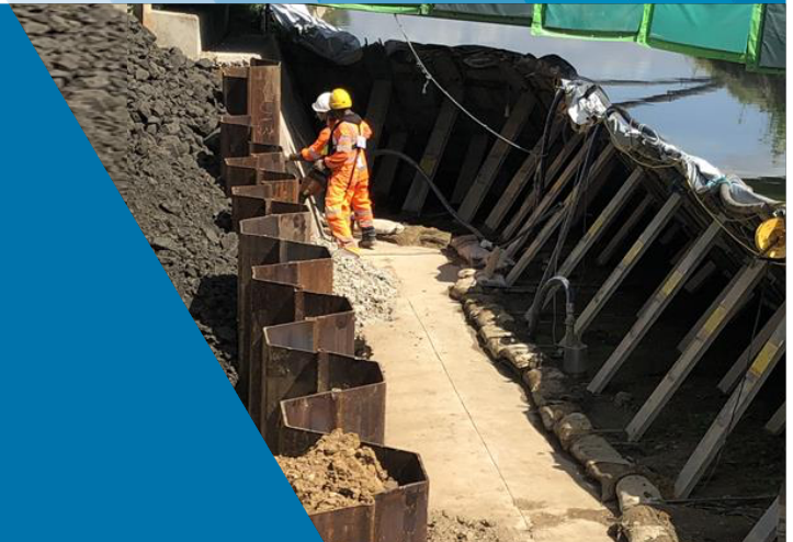
/// Breaking out existing concrete from bankside
