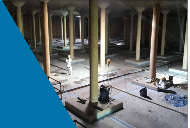
/// Internal works being carried out in the reservoir cell
